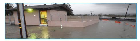
The Penngrove Lift Station Flood Resiliency project has been approved by the Sonoma Water Board of Directors. This project will elevate the Lift Station's electrical equipment out of the 500-year floodplain and will provide standby power to the station to allow operation during a storm.
